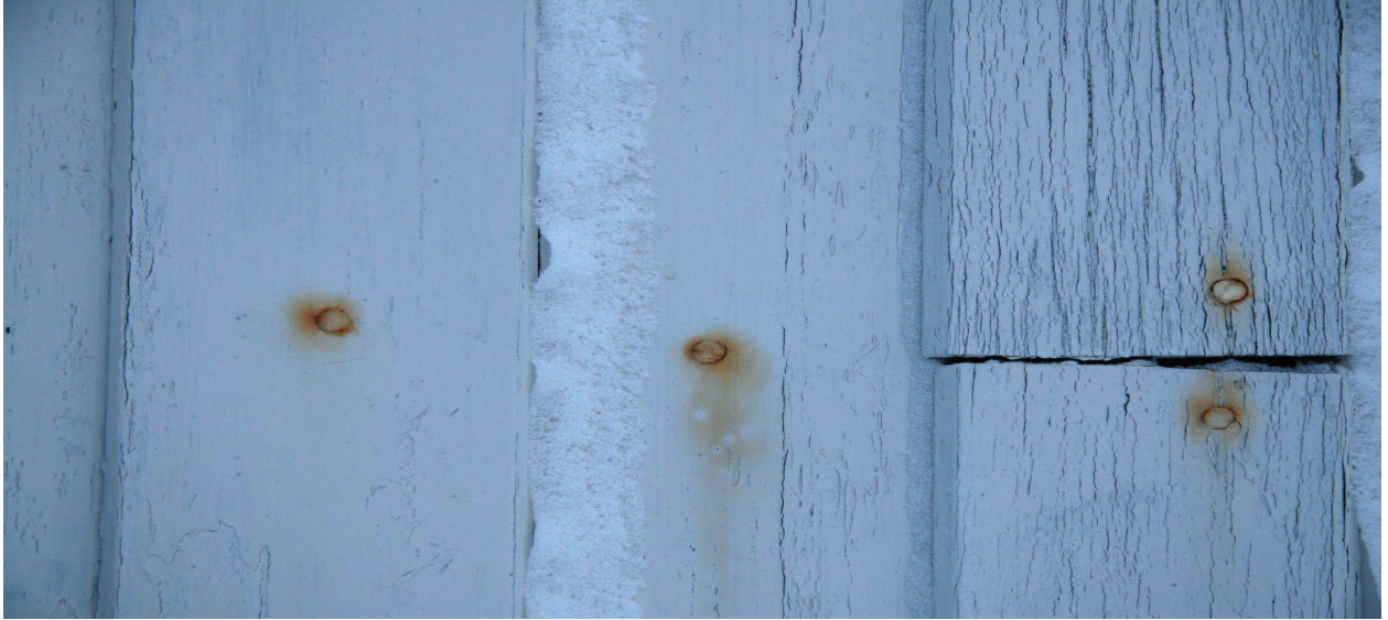
White fence, blue light, rusty nails
